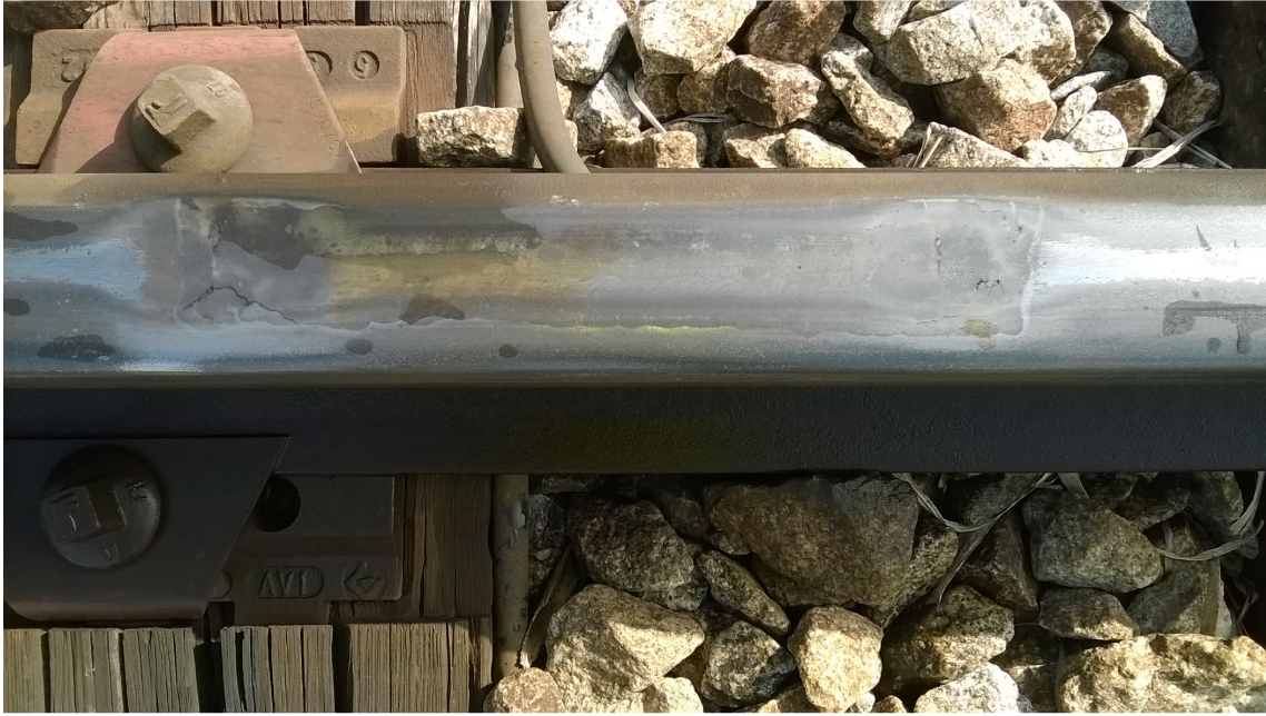
Figure 3 — Surface cracking
