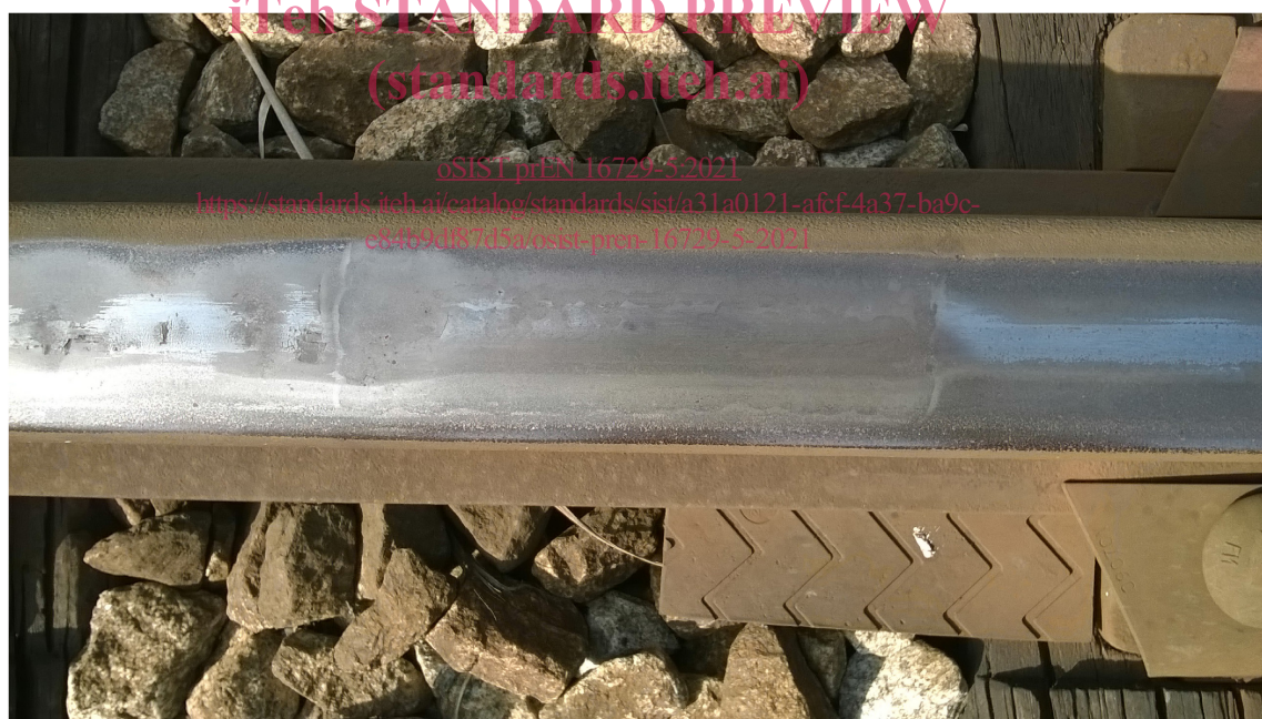
Figure 1 — Porosity on electric arc repair welds (a)
