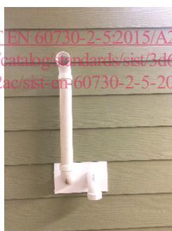
Figure 102 – Typical installation of the independent combustion air supply for room independent operation
