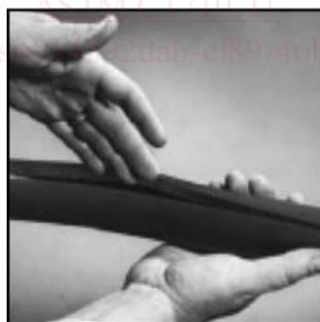
FIG. 3 Apply Unslit Insulation to Straight Pipe
