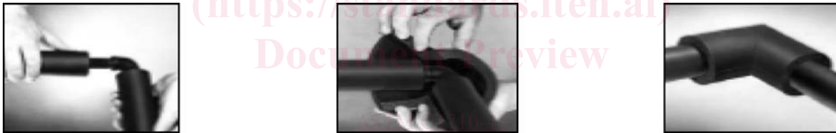
FIG. 6 Fabrication of Elbow
