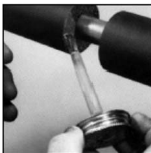
FIG. 2 Apply Adhesive to all Butt Joints Installed/Existing Pipe Work
