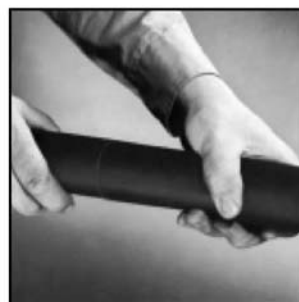
FIG. 2 Apply Adhesive to all Butt Joints Installed/Existing Pipe Work
