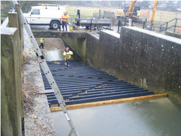
a) Baffles in the dry (viewed from upstream during construction)
