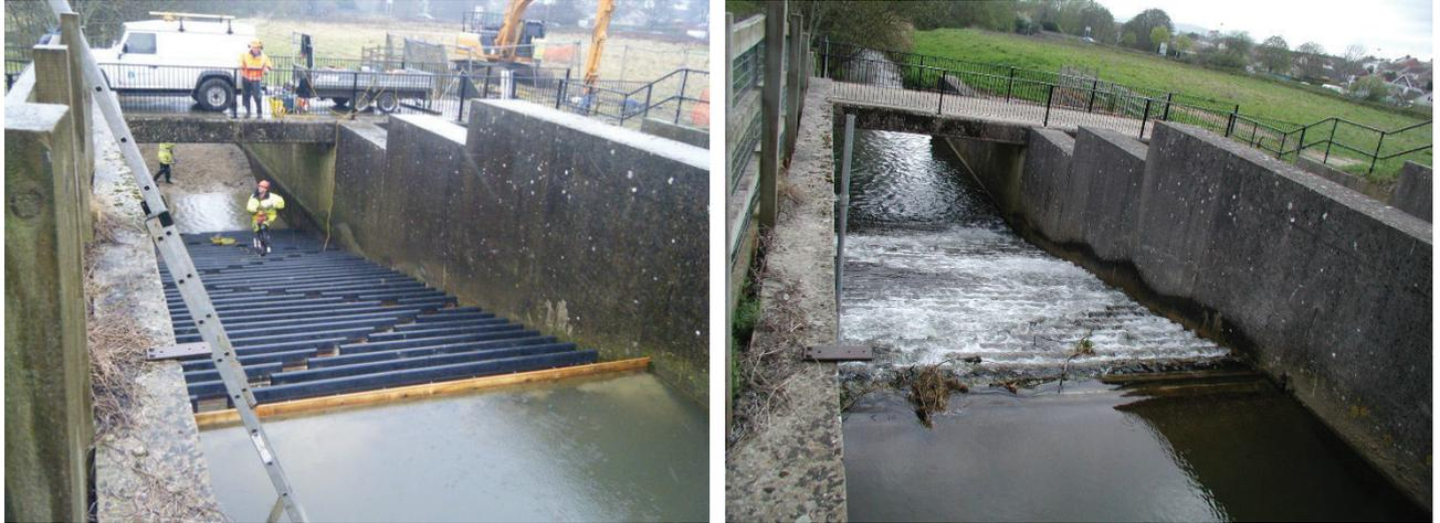
**a) Baffles in the dry (viewed from upstream during construction)**      **b) Baffles in operation before maintenance has been carried out (viewed from upstream)**
