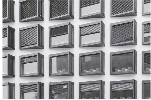
b) Windows with external venetian blinds. (Colour) photo by Samuel Zeller, CC0 1.0 DEED 2)
