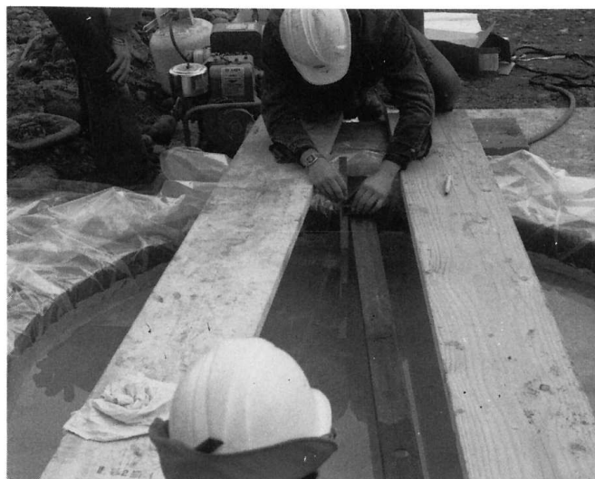
FIG. 3 Measuring the Water-Level Reference with a Carpenter's Square
