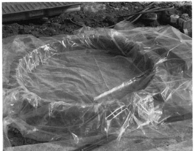
FIG. 2 Plastic Liner Placed in Preparation for the Initial Volume Determination
