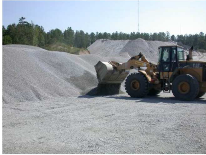
Step 2. Loader gently rolls the material out of the bucket to form a small pile
