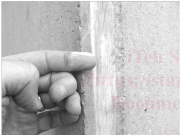
chalking, v—in building construction , formation of a powder on the surface of a sealant that is caused by the disintegration of the polymer or binding medium due to weathering.
