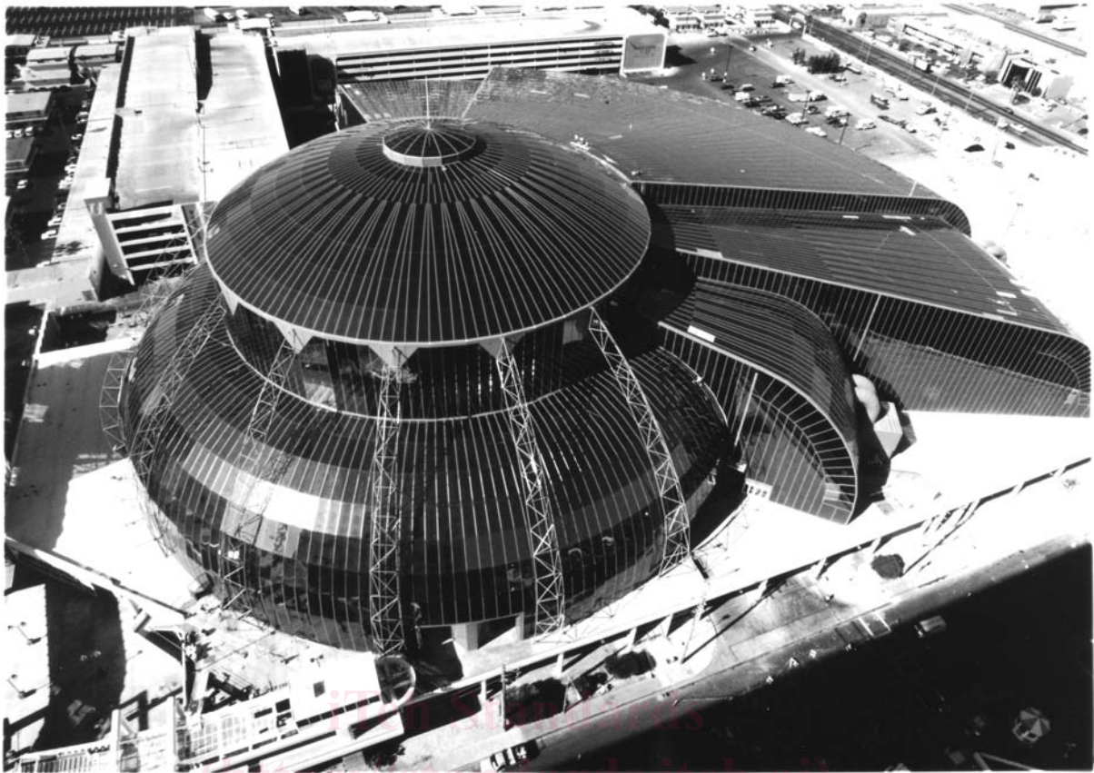
FIG. 5 Sloped SSG System
