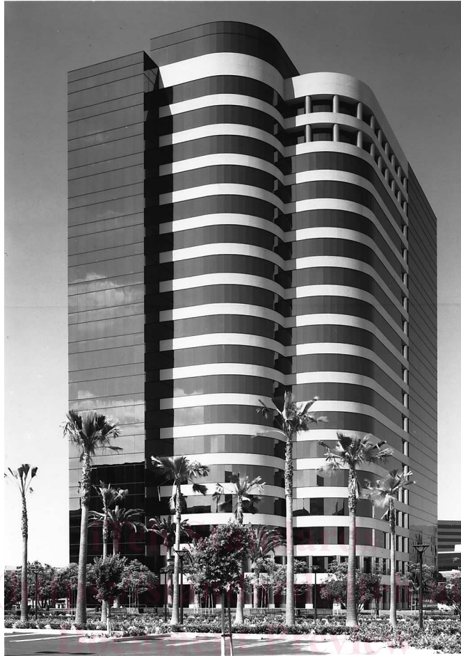
FIG. 2 Two-Side SSG System
