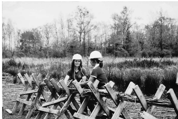
FIG. 1 Photograph of Live Fascine Fabrication (Tied Bundles, Not Installed)—Installed and Resting on X-Shaped Sawhorses)
