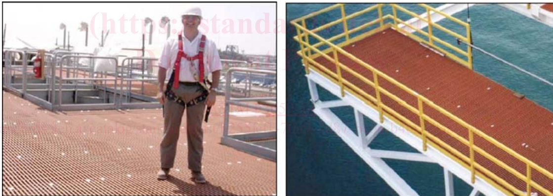
FIG. X1.1 Grating Floor Systems as Used Offshore
