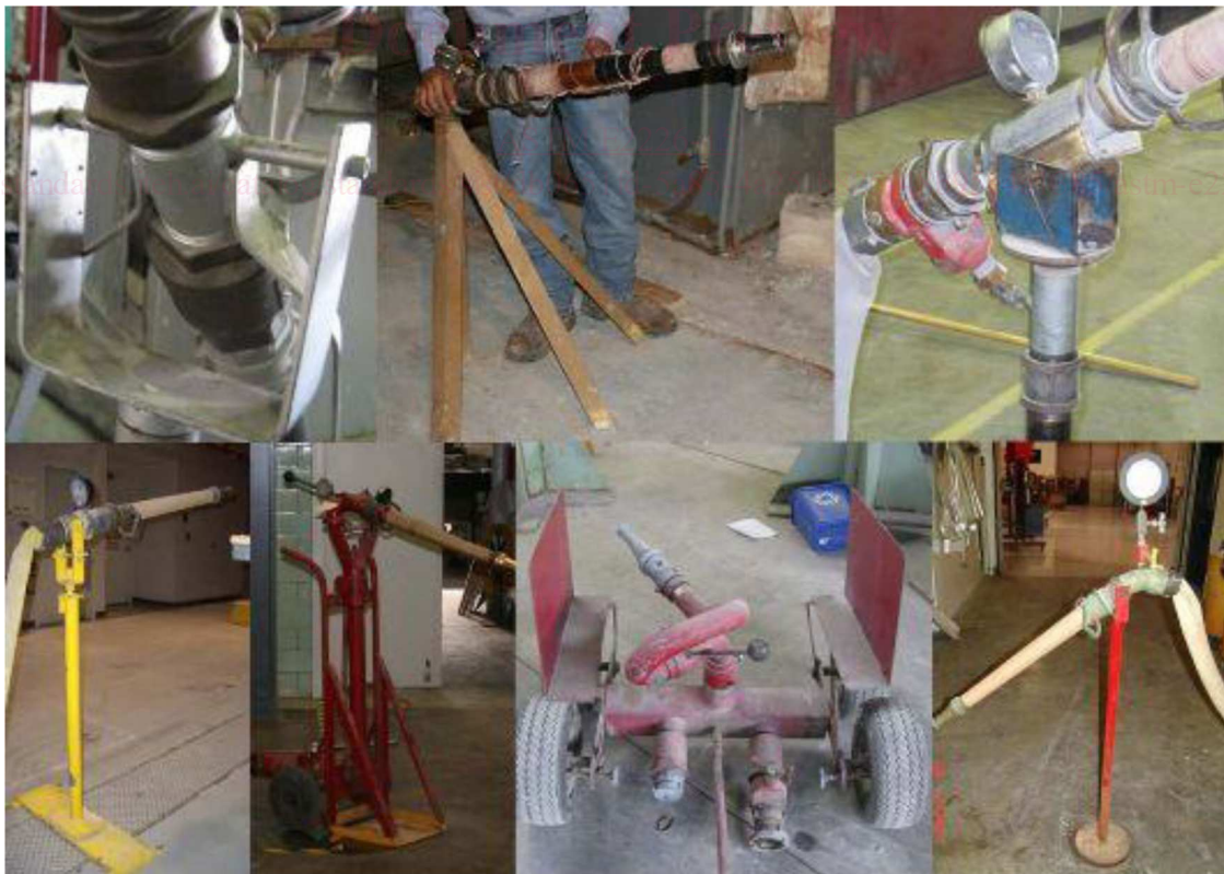
FIG. 2 Typical Hose Mounting Methods
