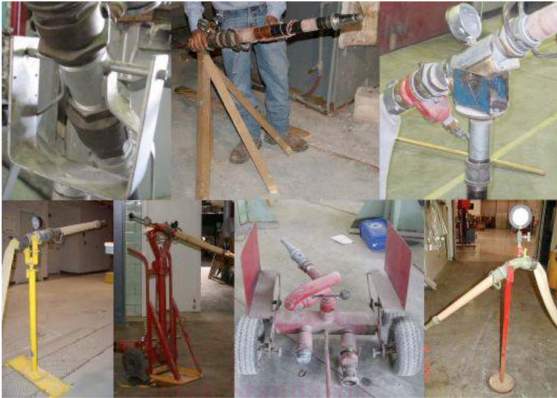
FIG. 2 Typical Hose Mounting Methods
