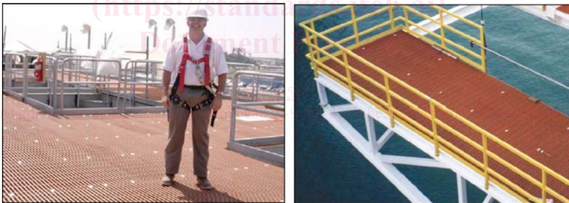
FIG. X1.1 Grating Floor Systems as Used Offshore
