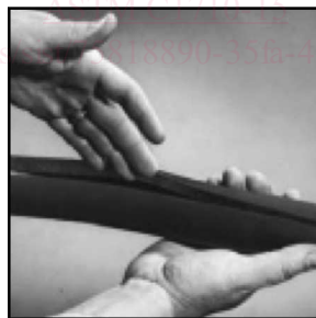
FIG. 3 Apply Unslit Insulation to Straight Pipe
