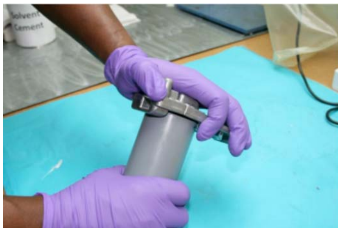
FIG. 7 Debur and Chamfer the Pipe End
