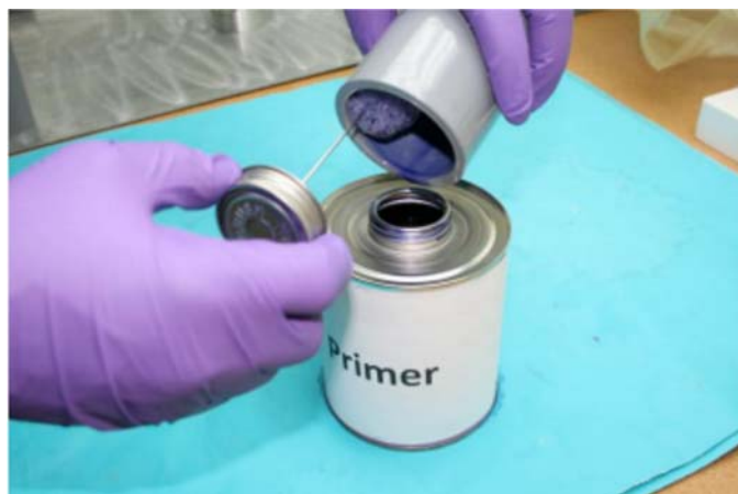
FIG. 11 Apply primer to the fitting socket.
