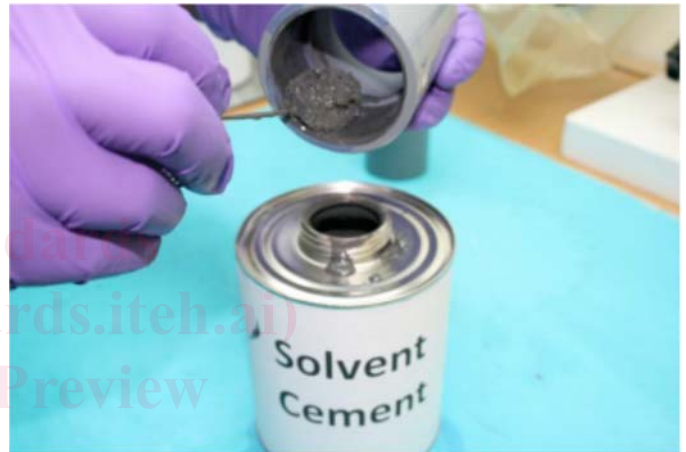
FIG. 14 Apply a thin and even layer of solvent cement inside the socket.
