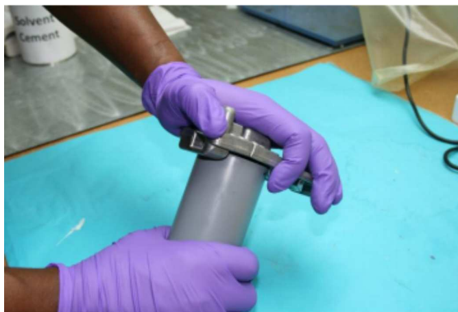
FIG. 7 Pipe Entering Dry Fitting
