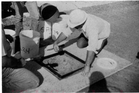
FIG. 5 Excavation of the Test Pit
