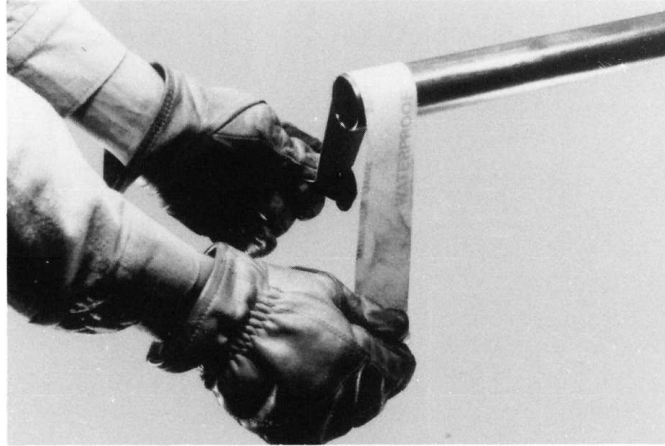
FIG. 6 Cleaning: Sand Cloth
