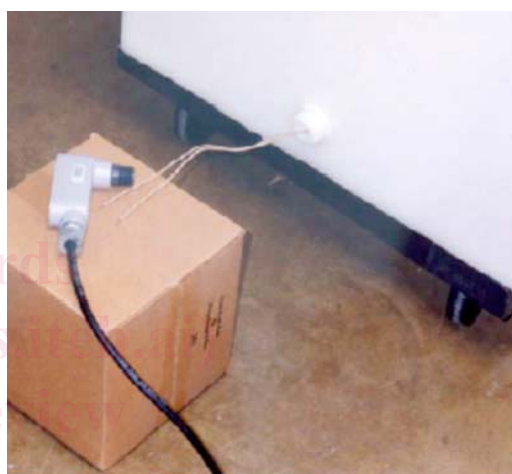
FIG. 7 TC Heater Installed in Tank Exterior
