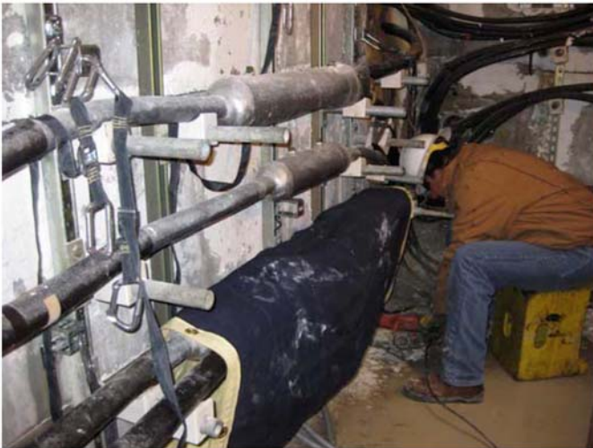
FIG. 3 Blanket Installation (clamshell method over cable splices)
