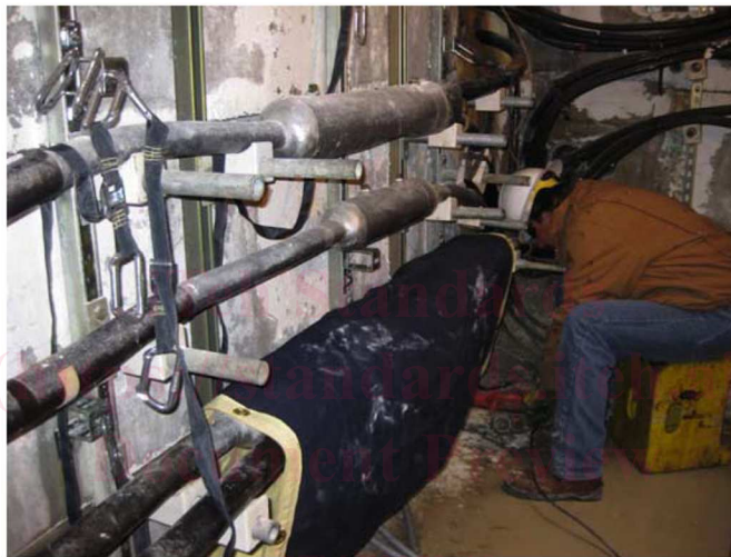
FIG. 3 Blanket Installation (clamshell method over cable splices)
